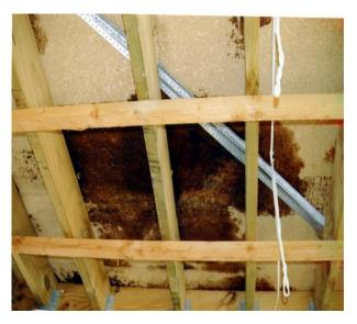
The photograph on the left shows the effects on an area subjected to wetting, which was floored with ordinary particleboard and insufficiently protected with a poorly applied membrane.
